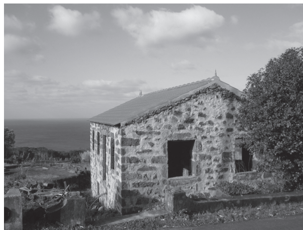
Figure 3: The ruin acquires a roof.
