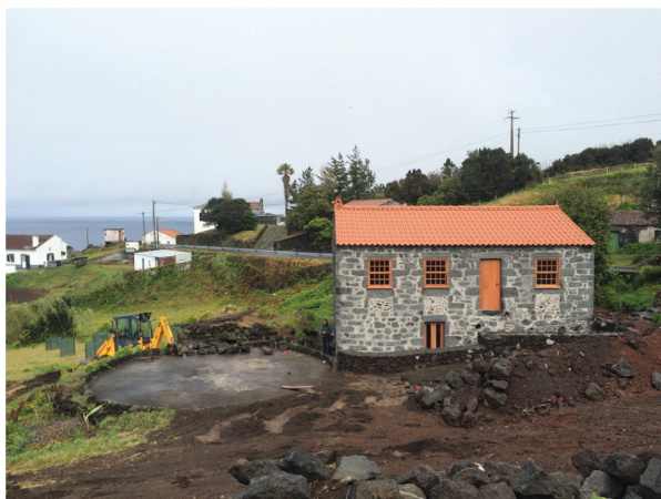
Figure 1: The former ruin, now a house with roof, doors, and windows.
